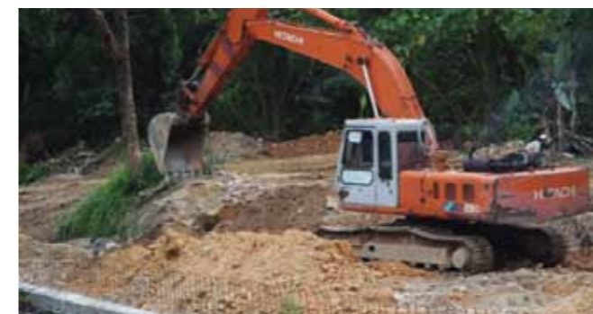
Flood mitigation work behind Taman Tunku
