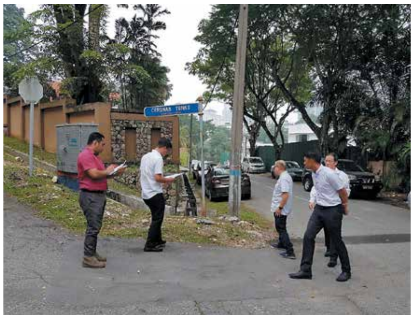
Joint inspection by BTRA Environment Sub-Committee and DBKL officers of street and drain conditions at the junction of Dalaman Tunku and Cerunan Tunku
